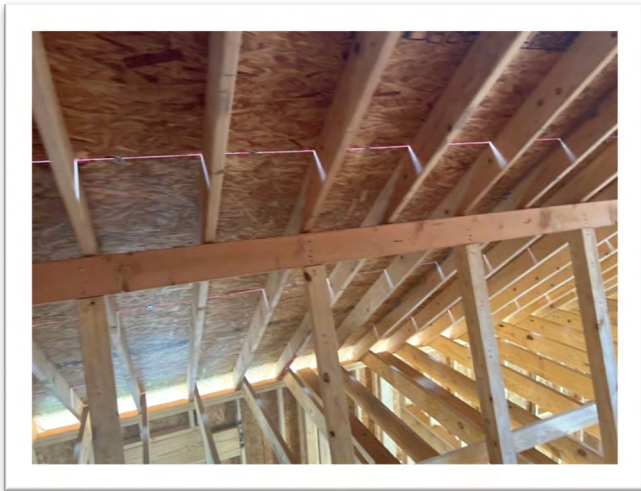
Attic Rafter Photos
