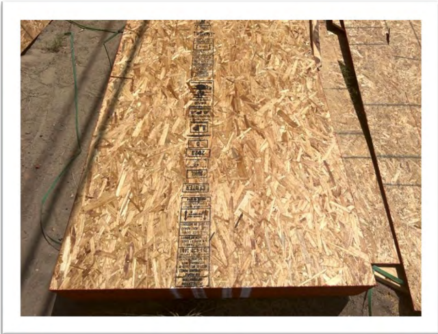
Roof Deck Thickness
