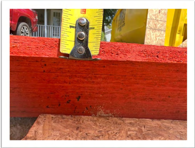
Roof Deck Thickness
