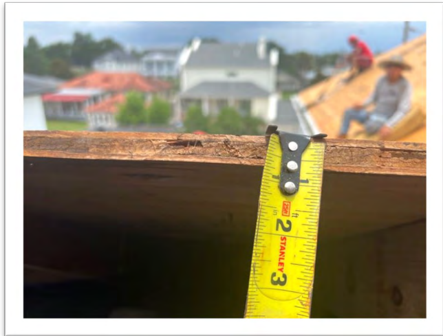
Roof Deck Thickness
